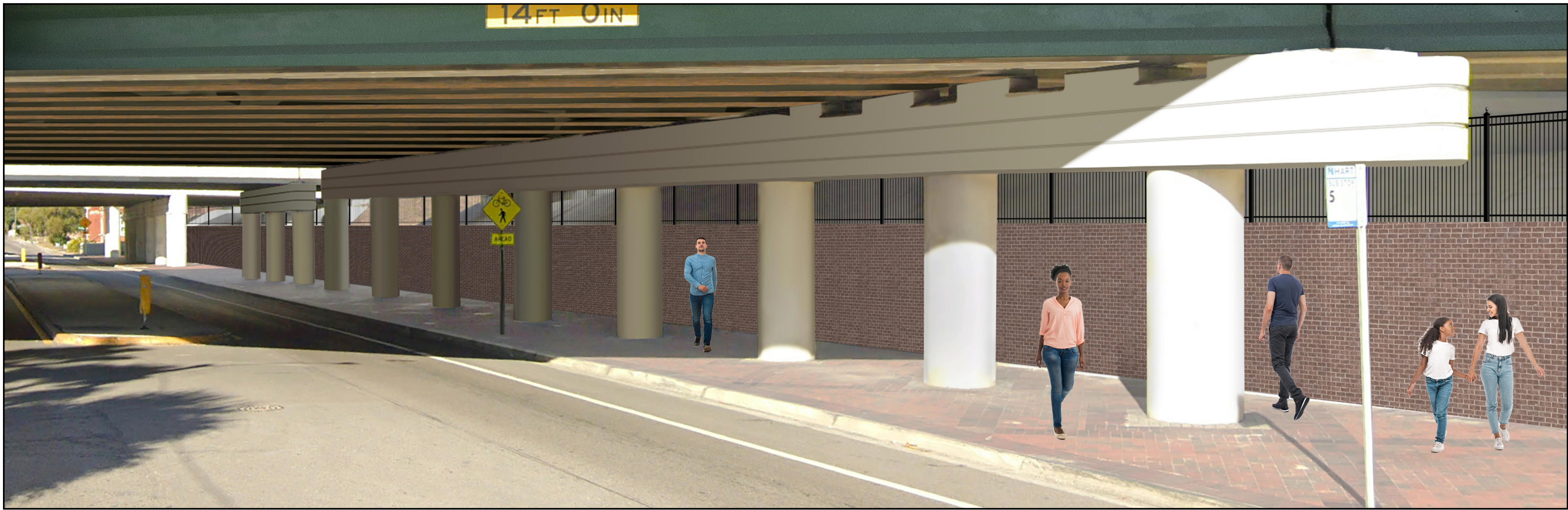
Palm Avenue - brick facing on gravity walls
