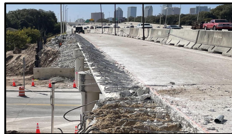
Removal of Barrier Wall and Bridge Deck
